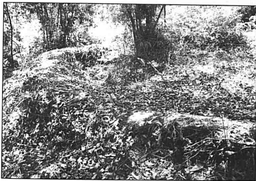
'Vickers Machine-gun position' providing ample protection against Japanese planes low-level strafing-This bunker is located on Green Ridge.
